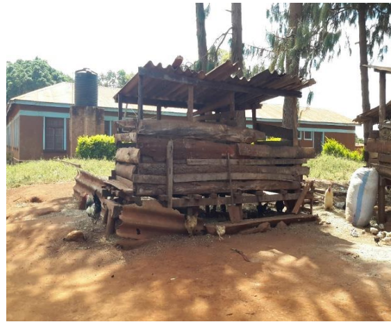
FIGURE 4d: Misheni Street (Mbinga District)
